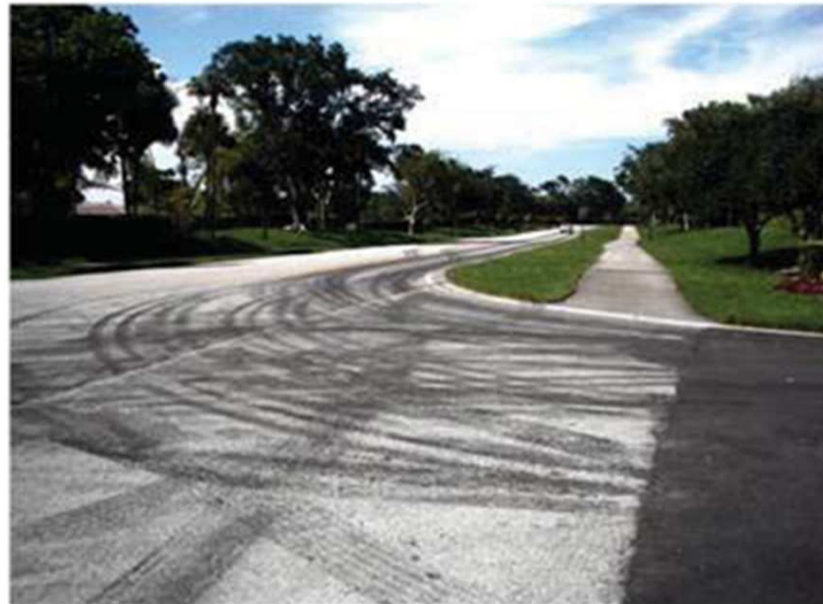
Tracking from Conventional Tack Coat
