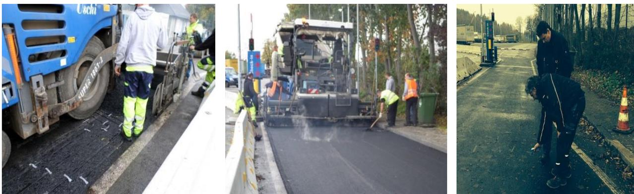
**Figure 12: Applying the top asphalt layer**
