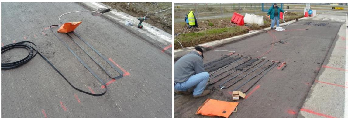
**Figure 14: Ribbon serpentine installation**
