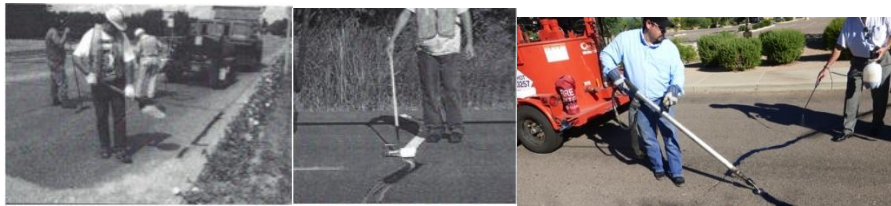
Figure 22: Blotter Applications
