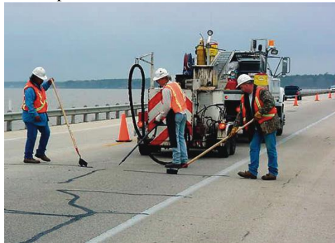
Figure 23: Crack Treatment Operations (31)
