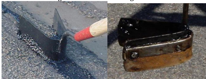
Figure 8 : Squeegee for Sealant ((A)Hot Poured Sealant on left, (B)Cold Poured Sealant on Right) (31)
