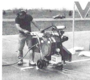
Figure 12: Diamond Saw Crack Cutting (35)
