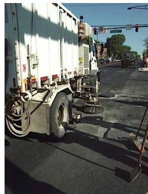
Figure 14: Pavement Sweeping (Photograph by Dale Decker)
