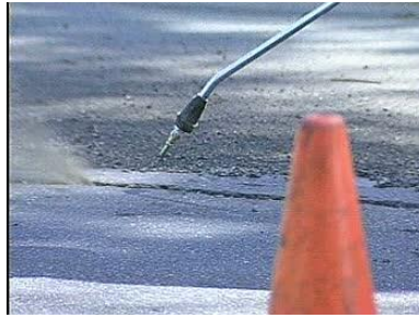
Figure 15: Compressed Air Cleaning of Crack (Courtesy Crafcoc)
