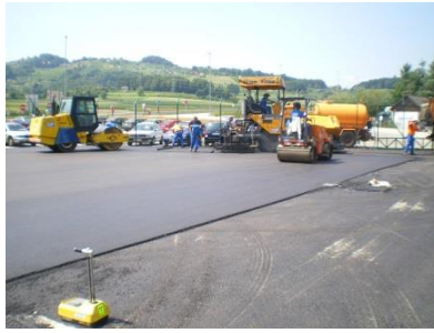
Figure 3: Construction of test field with PMMA/ATH composite dust in wearing course in 2009 (a.) and the same test field in 2013 (b).
