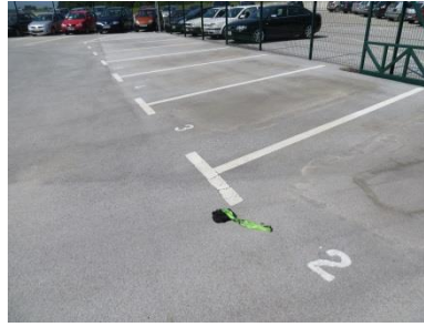
Figure 3: Construction of test field with PMMA/ATH composite dust in wearing course in 2009 (a.) and the same test field in 2013 (b).
